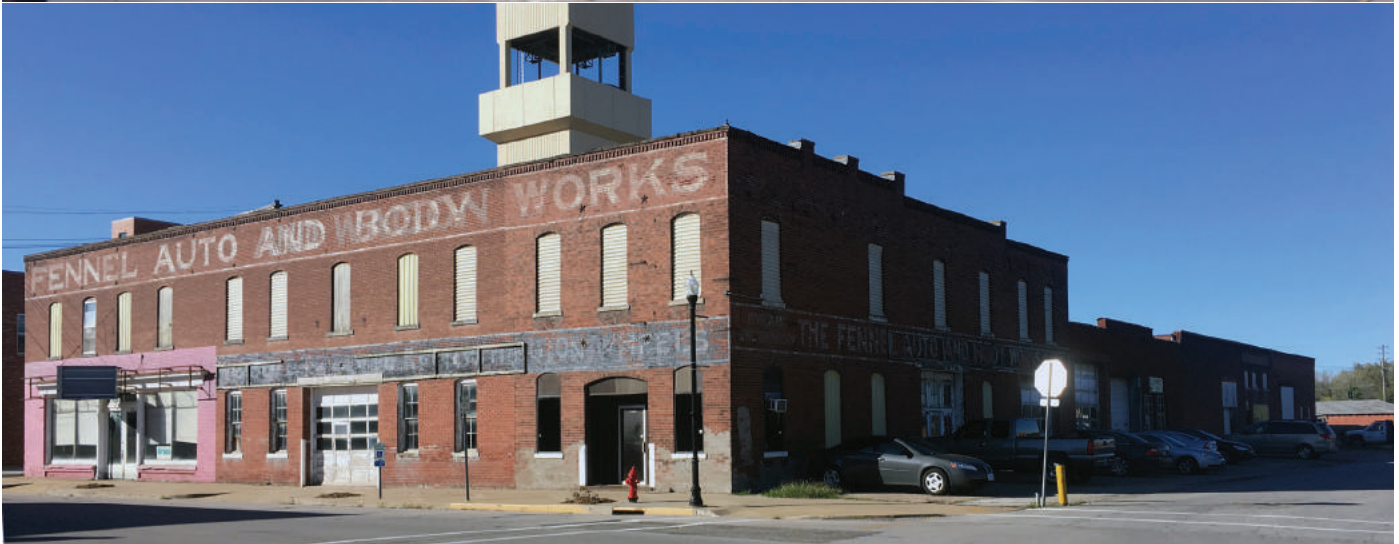
The Fennel Auto building has had its masonry altered throughout time in various ways, such as tuckpointing, painting, the filling in of old windows, and punching new openings. This causes the current facade conditions shown in the bottom image to look like a non-uniform “patchwork” of alterations. Acceptable treatments to this building are such that when the mortar is damaged it should be tuckpointed in those damaged areas but nowhere else.
