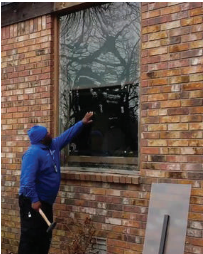
Clear polycarbonate sheeting board is the preferred window covering for existing windows in downtown Moberly.
